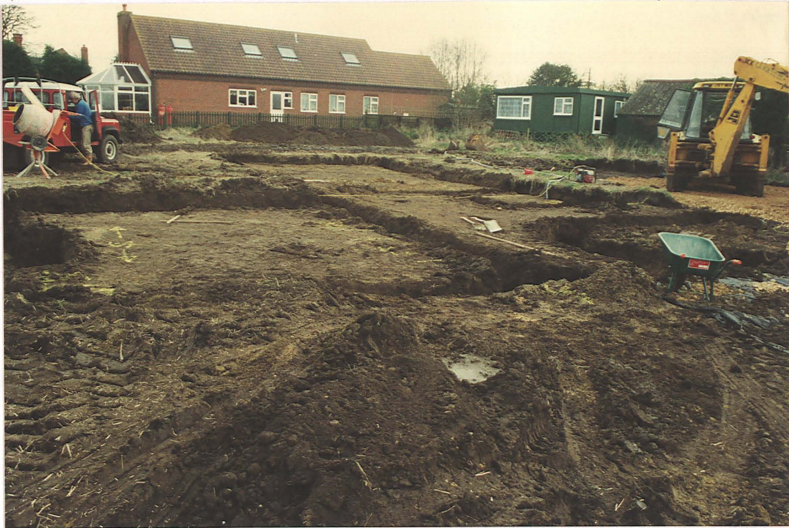
Pl. 5 The plot after excavation of foundations of the proposed building.
