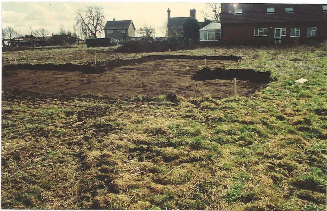
PI. 4 The site after partial topsoil removal looking south-east.
