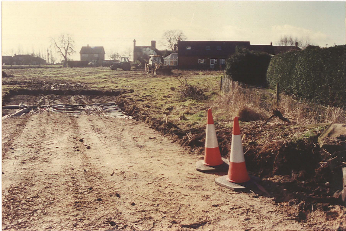
PI. 1 The site prior to excavation looking south-east away from Church Lane.
