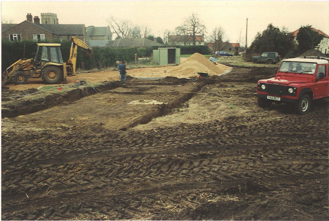
PI. 3 Excavation of foundation trenches under archaeological supervision looking north-west.
