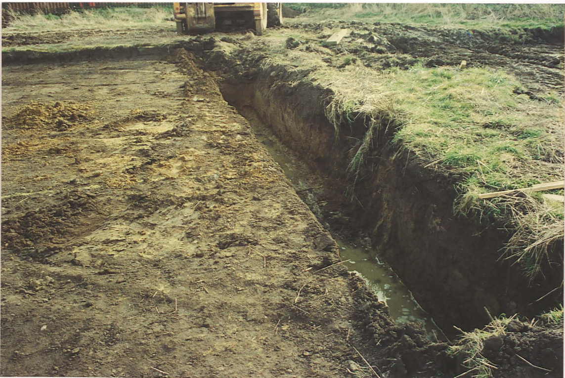
Pl. 6 Foundation trench, note in the foreground feature 104, looking south-east.
