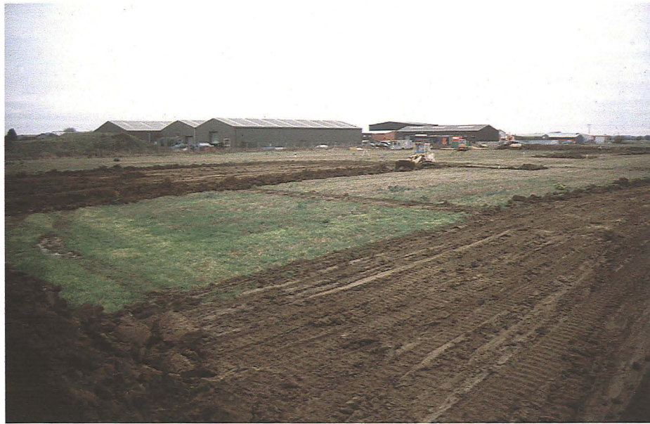
Plate 1 General view of development area during initial site strip, looking northwest.
