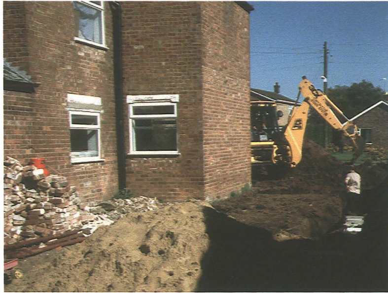
Plate 1 General view of site during groundworks
