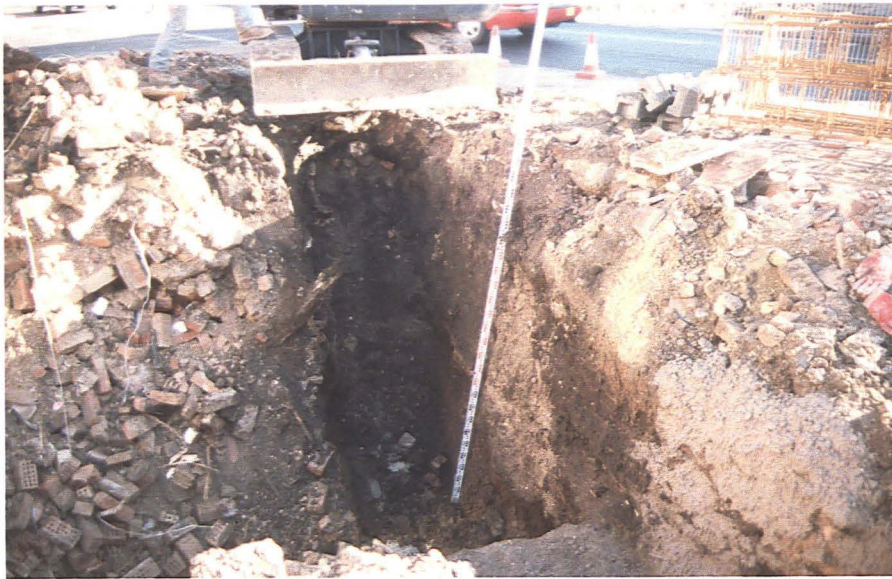
Plate 1 Working shot of excavation of footings, looking southeast.
