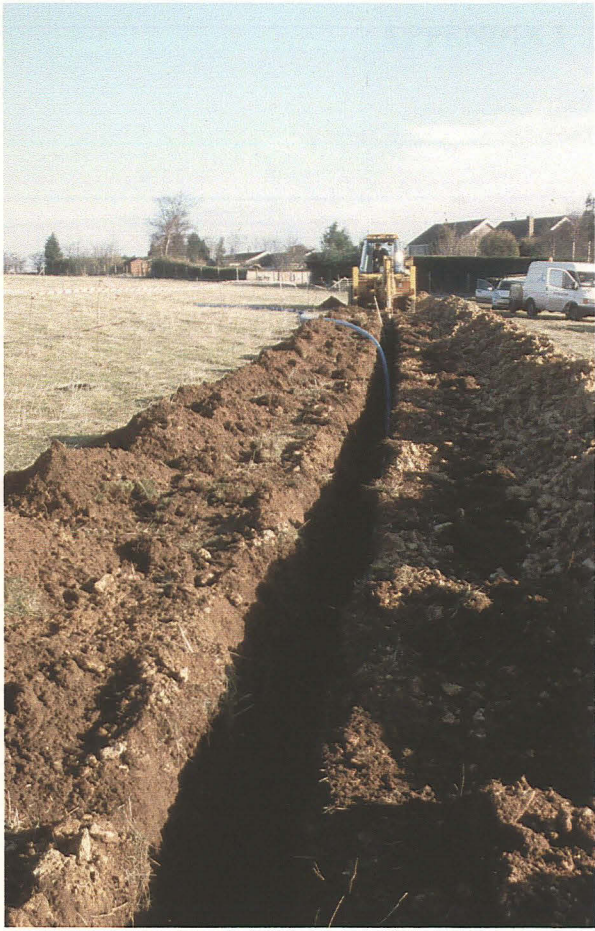
Plate 1 General view of site during excavation of pipe trench, looking northeast.
