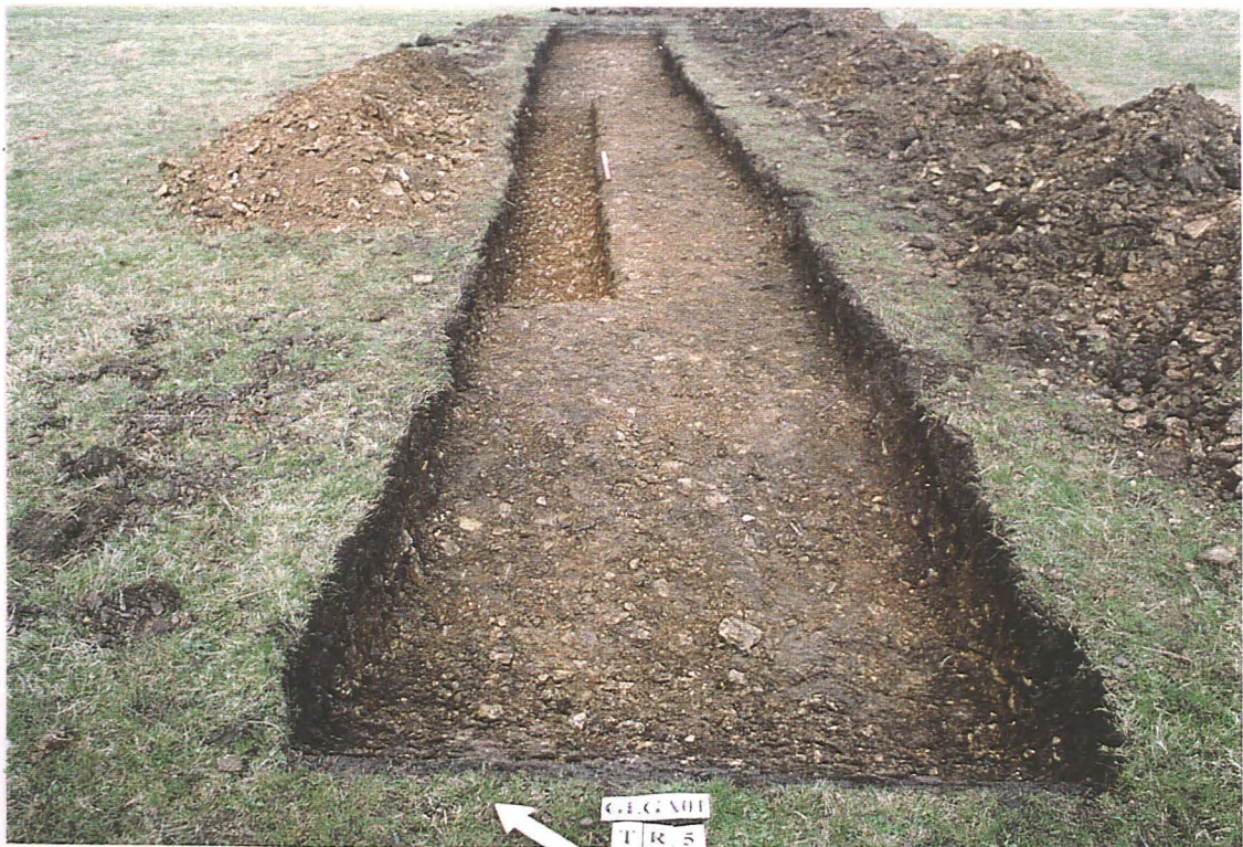
PI10: Post excavation shot, Trench 5, looking north-east
