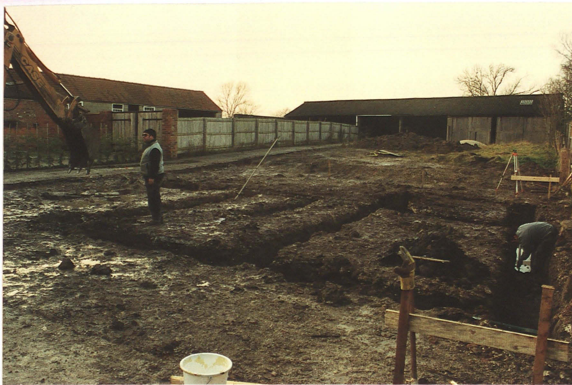
Pl. 3 The new house foundation trenches, showing the sloping ground (looking NW).
