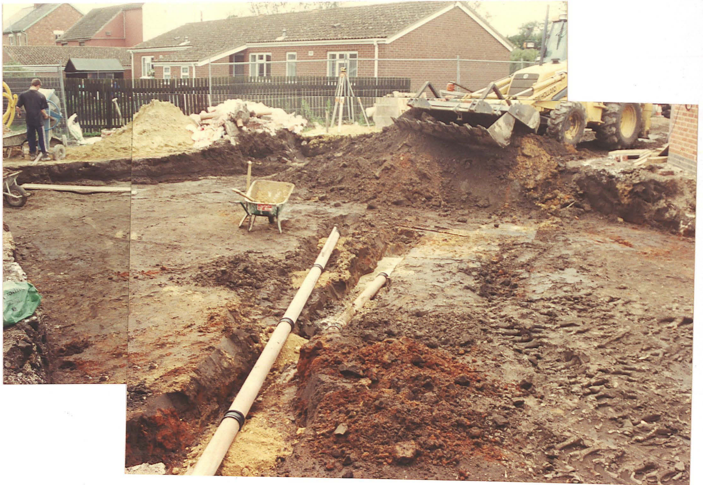
Pl. 6 Service trenches across the access road (looking SW).
