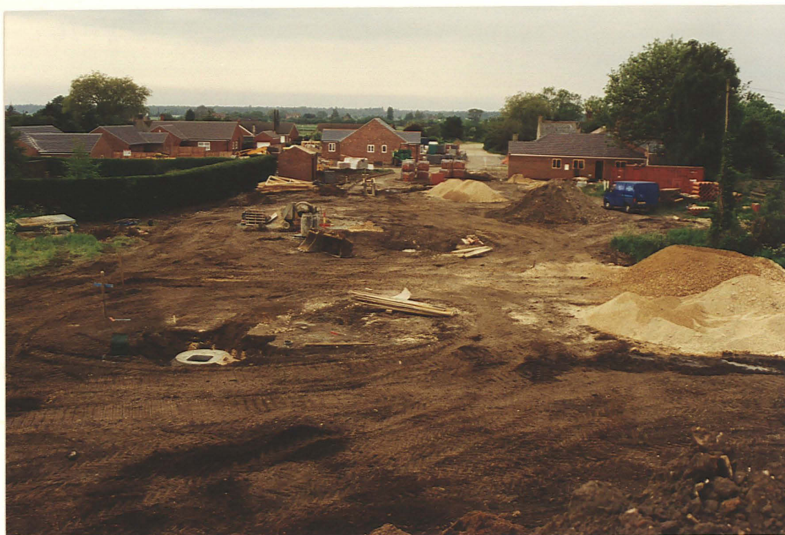
Pl. 1 View of the site during development (looking west towards Watery Lane). The manholes mark the line of the west-east sewer trench (backfilled), with the manhole in the foreground coinciding with the fork in the access road. The electricity sub-station is beside the hedge, centre left.
