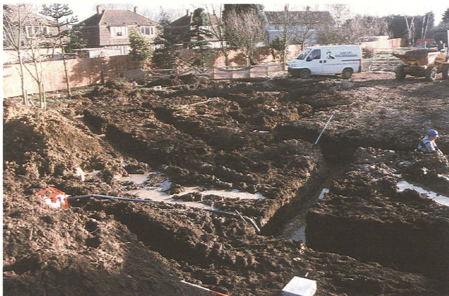
Plate 1 General view of site after completion of footing, looking southeast.
