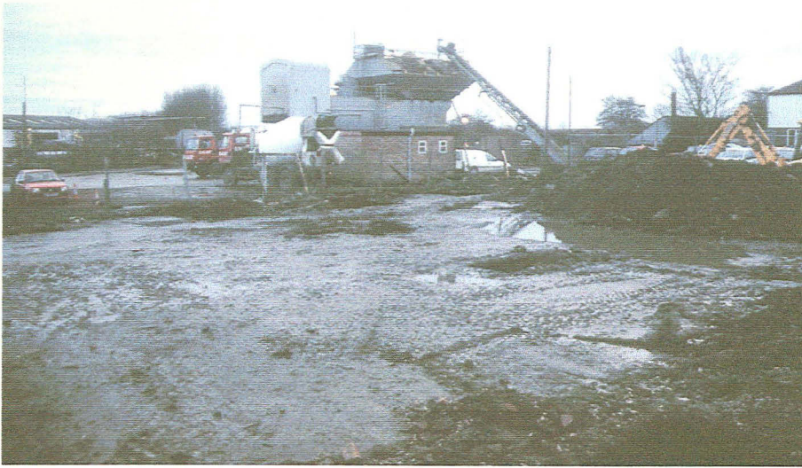
Plate 1 General view of site during groundwork, looking east.
