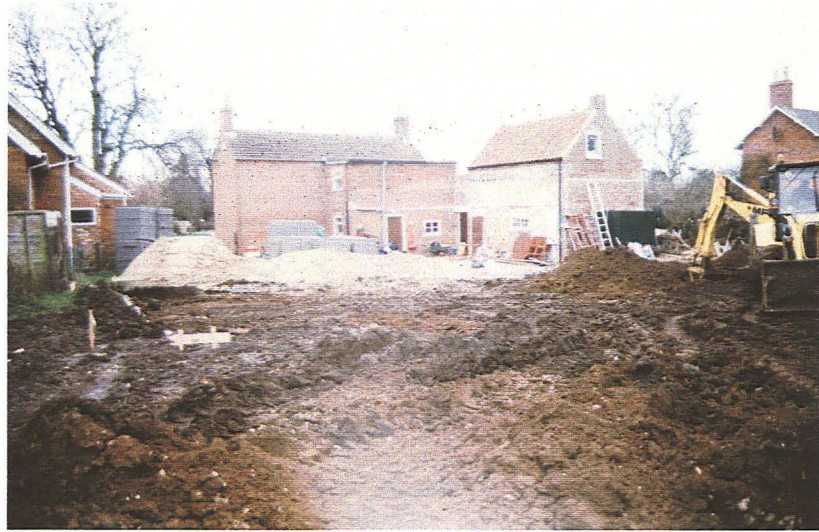
Plate 1 - General view across the development area, looking south
