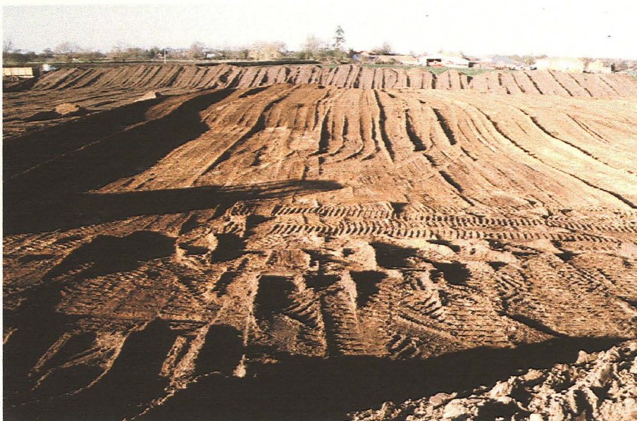
Plate 1 General view of site during excavation, looking north.
