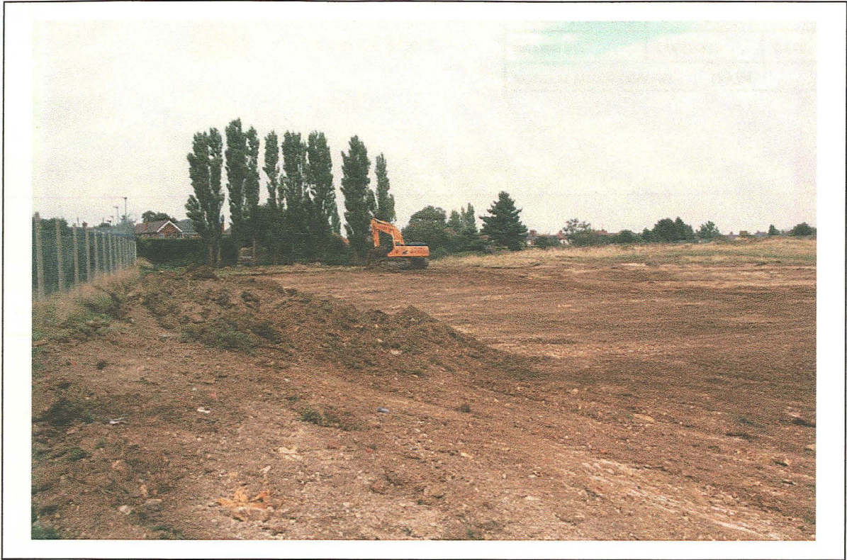
Plate 1: General view of topsoil stripping in progress - looking north
