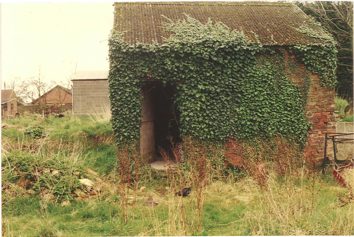
Pl. 8 Small brick shed in the centre of the site; note the blocked circular hole to the right of the ivy (looking south).
