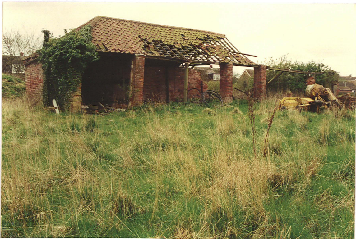
Pl. 7 Open-fronted brick sheds in the centre of the site, near the western boundary (looking SW).
