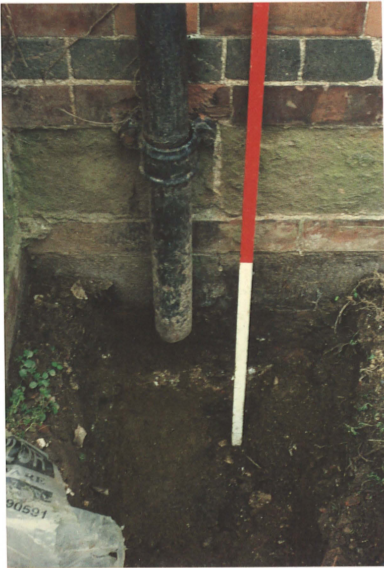
Pl. 4 Trench 3, Looking north showing top of stepped foundations and backfilled test pit from 1998 evaluation. Scale 1m.
