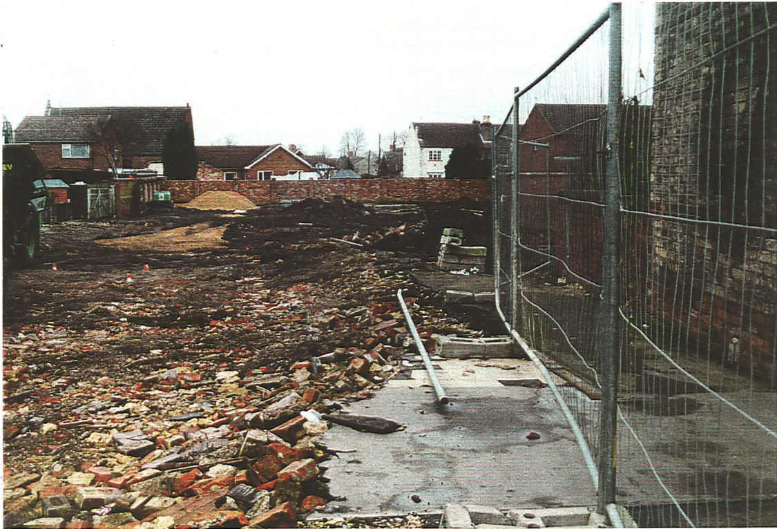
P1: General view of the site, looking north
