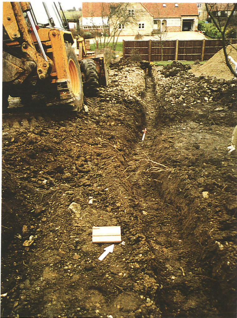
Pl. 2. Detail of service trench excavations, looking NW.
