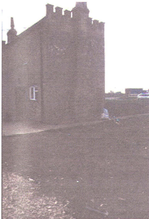
Plate 1 - General view of the western area of development, looking southeast
