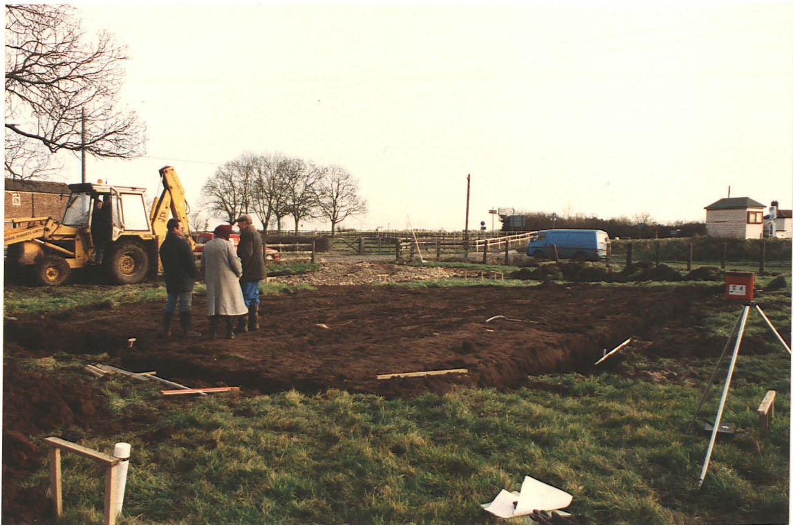
Pl.2 Excavation of foundations looking north east towards by-pass.
