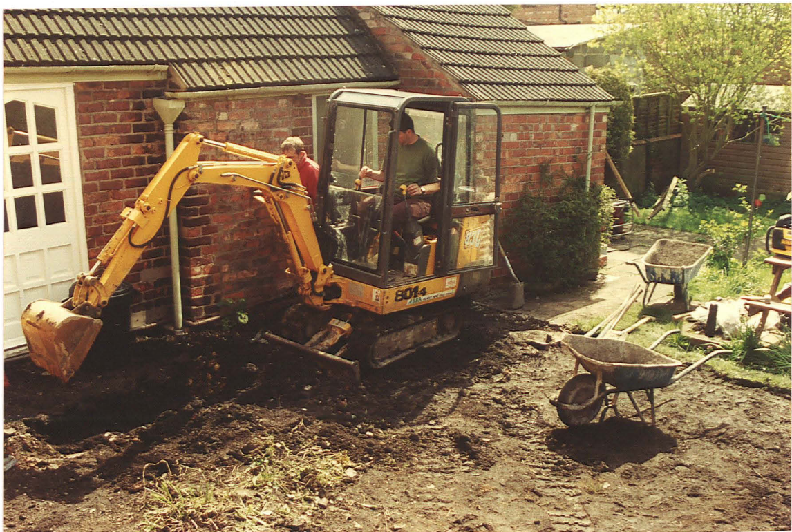
Pl. 2 Machine excavation of the extension footings.
