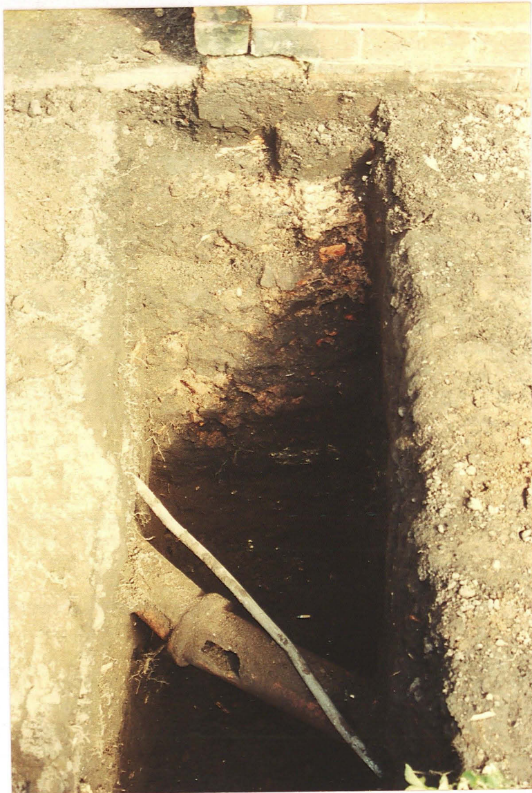
Pl. 3 Depth of house footings mark the depth of made up ground.
