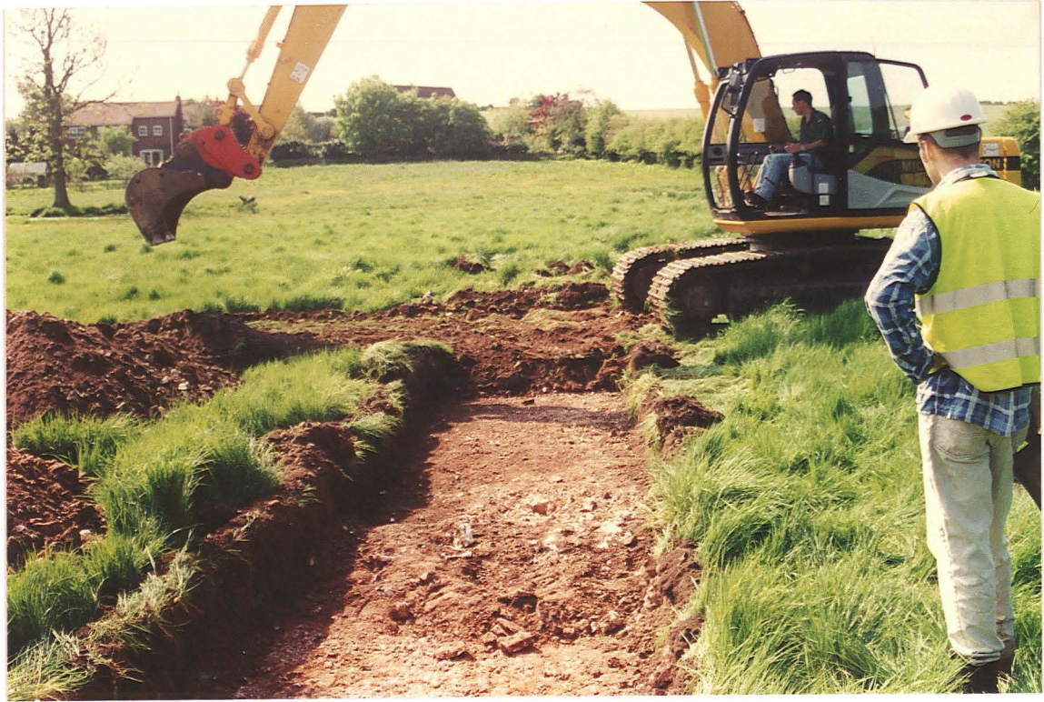
PI. 2 Machine excavation of trench under archaeological supervision.
