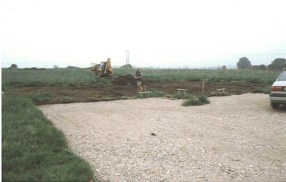
Plate 1 General site view, looking southeast
