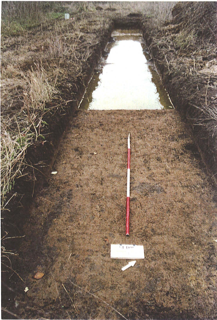
Plate 9: Trench 03 after machining, looking north-west.
