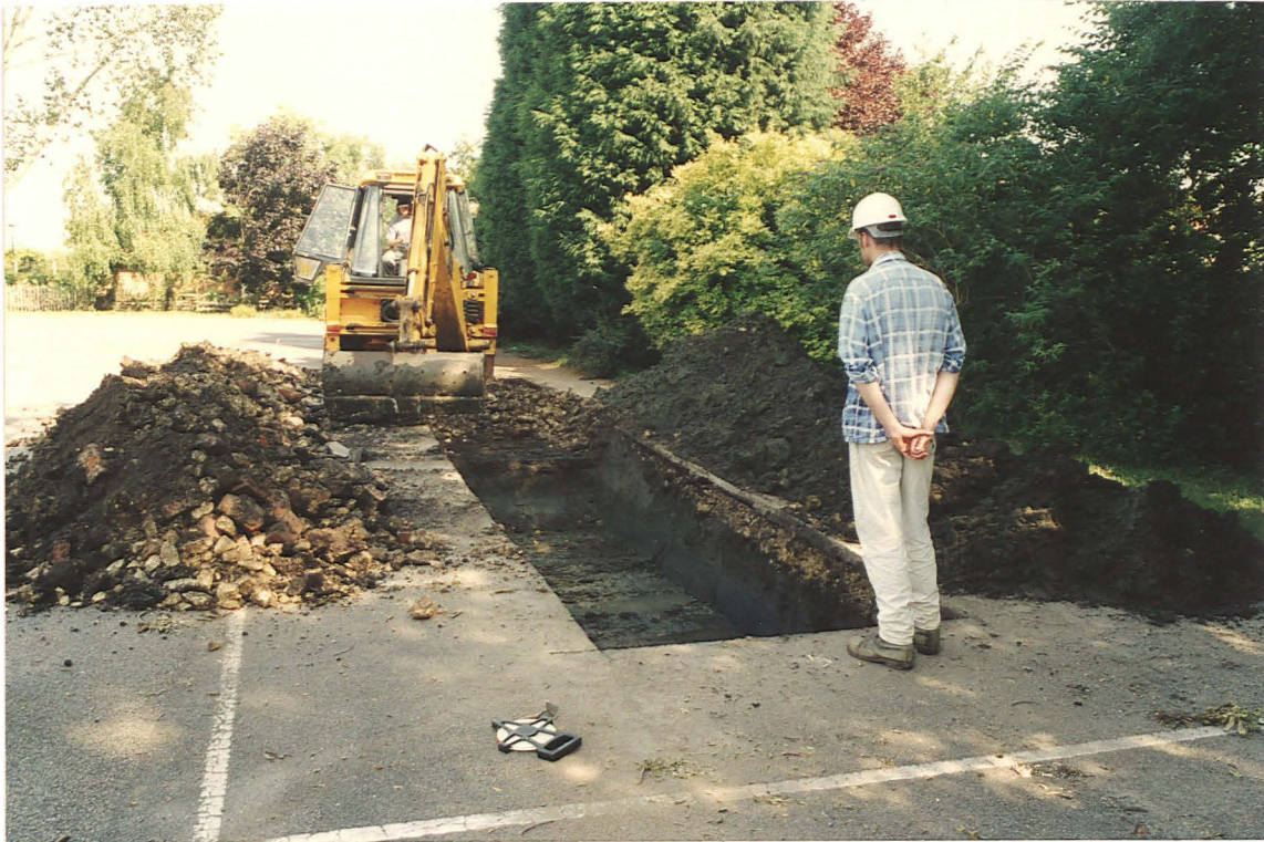
Pl. 1 Machine excavation of Trench 2 under archaeological supervision.
