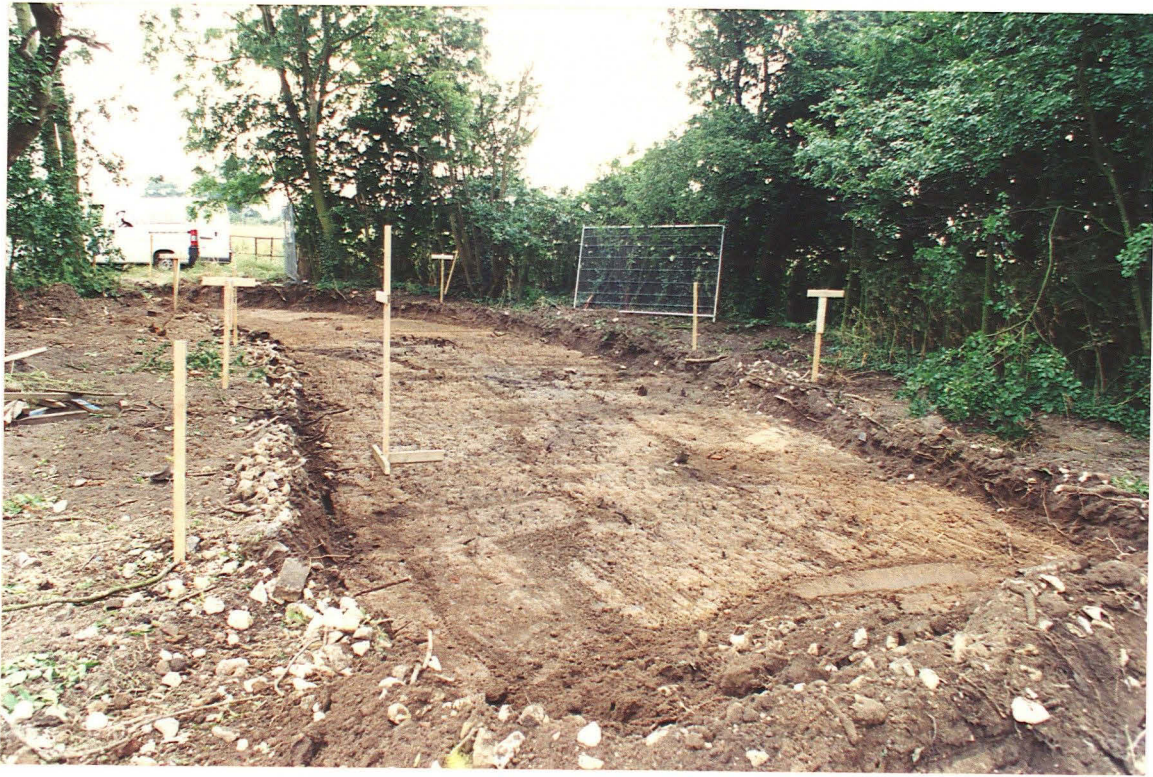
Pl. 3 Access road looking south
