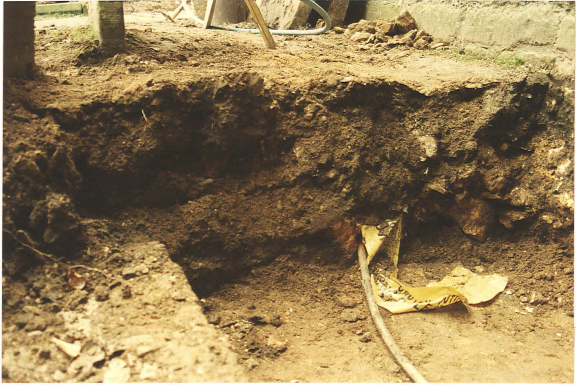
Pl. 2 West facing elevation, showing foundation stones beneath north aisle west wall.
