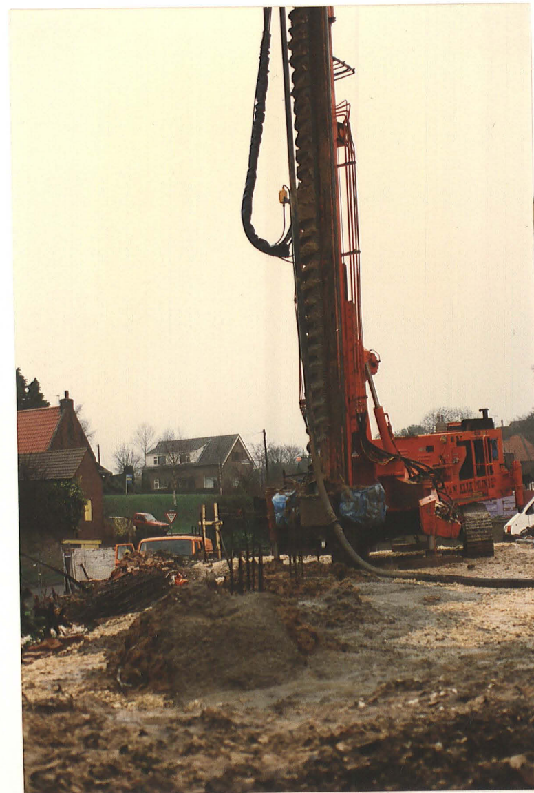
Pl. 13 Auger arm of Soilmec drilling rig showing concrete feed hose attachment at top centre of auger
