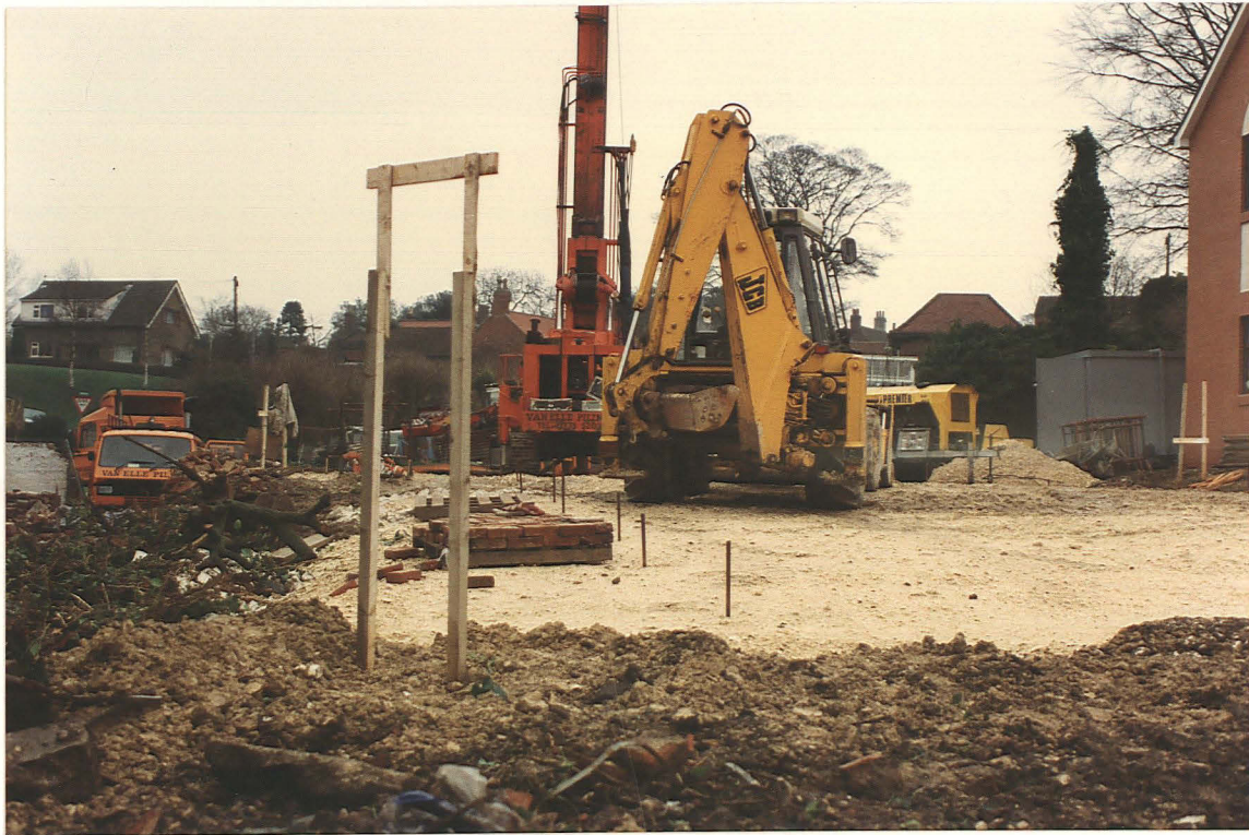
Pl. 11 Phase 2 site, view E. Stakes mark piling positions
