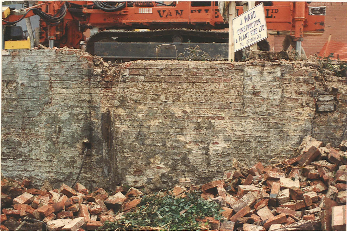
Pl. 5 Demolished barn S wall, internal elevation showing example of blocked openings
