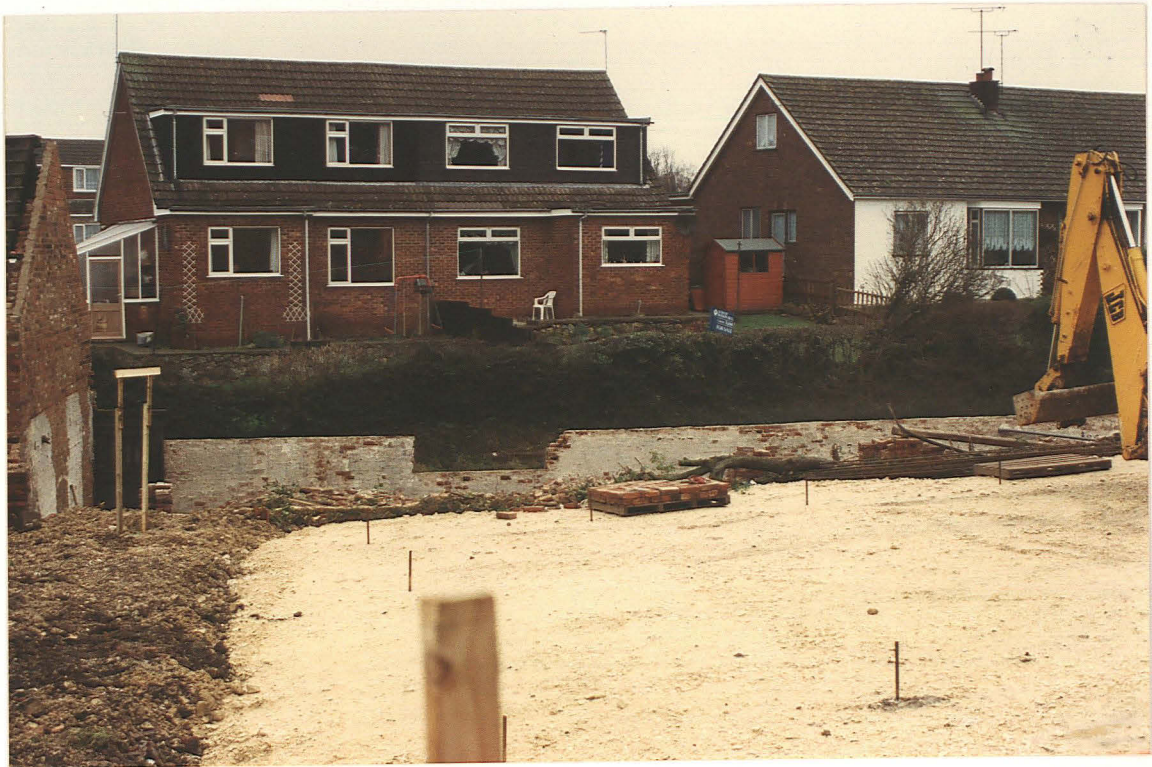
Pl. 9 NW corner of Phase 2 site, looking N. Stakes mark piling positions
