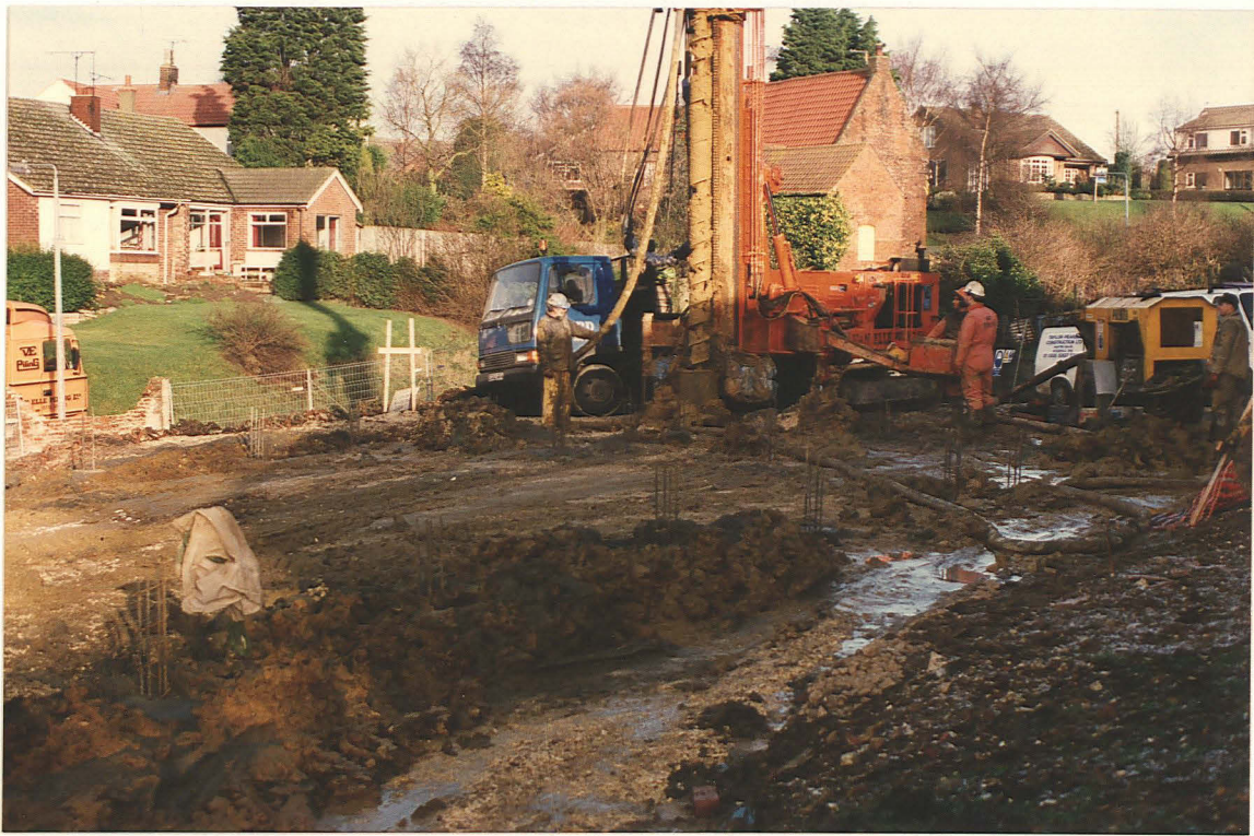
Pl. 19 Drilling in progress at NE corner of site
