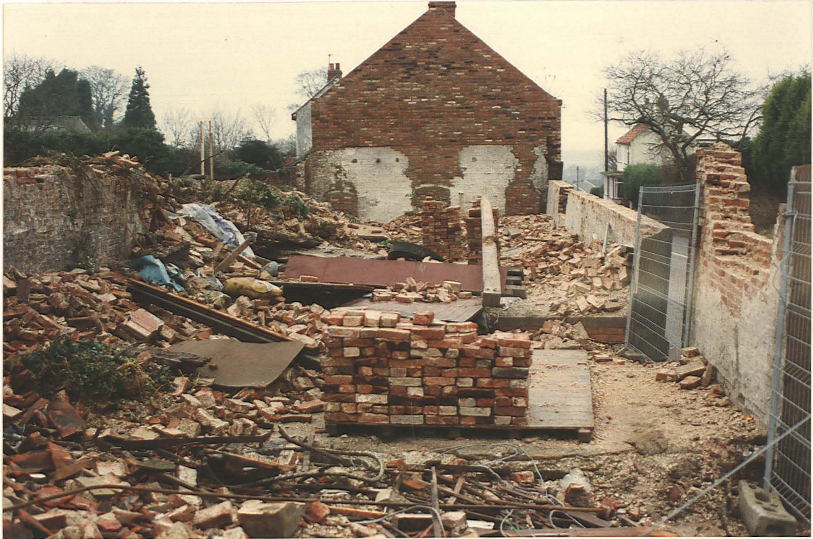
Pl. 3 Demolished barn showing varying concrete floor levels
