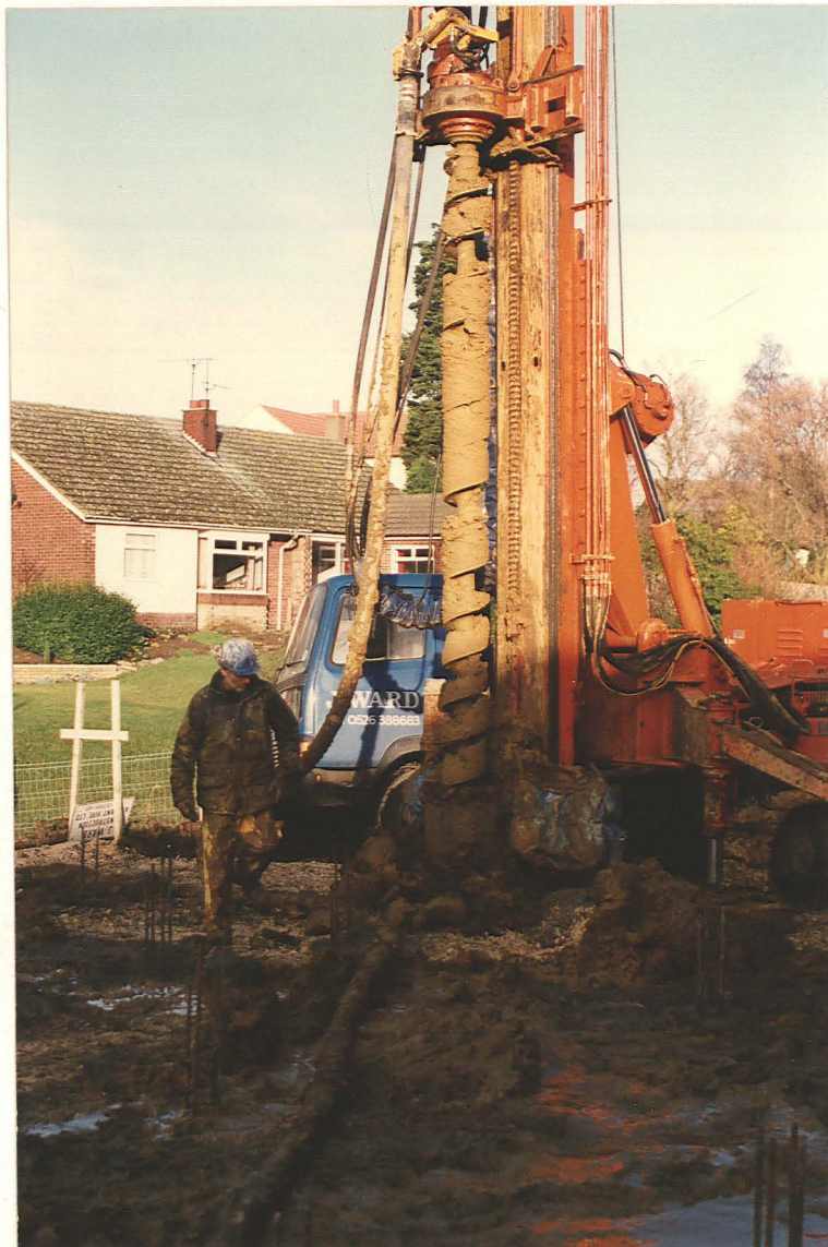
Pl. 20 Drilling in progress at NE corner of site
