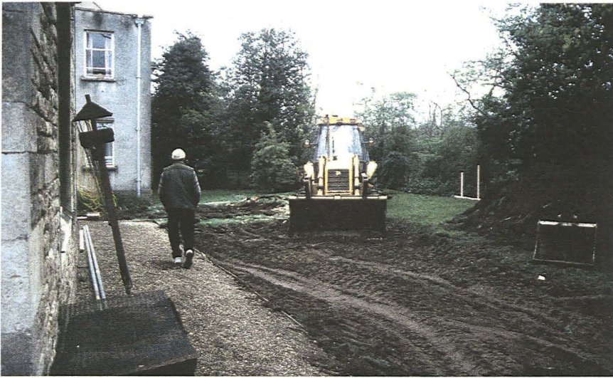
Plate 1 General view of topsoil stripping, looking east
