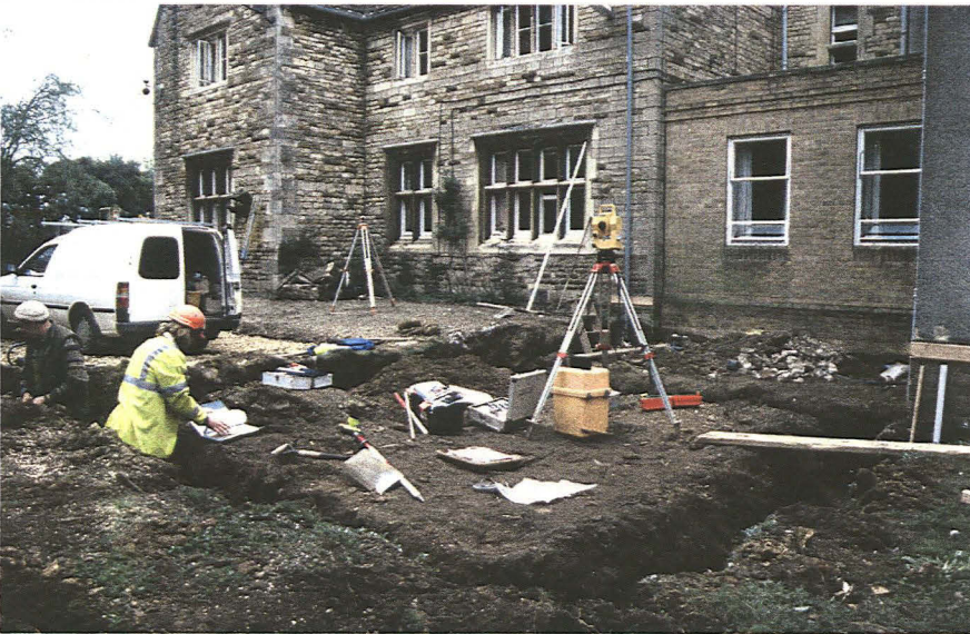
Plate 2 General view of work in progress, looking northwest
