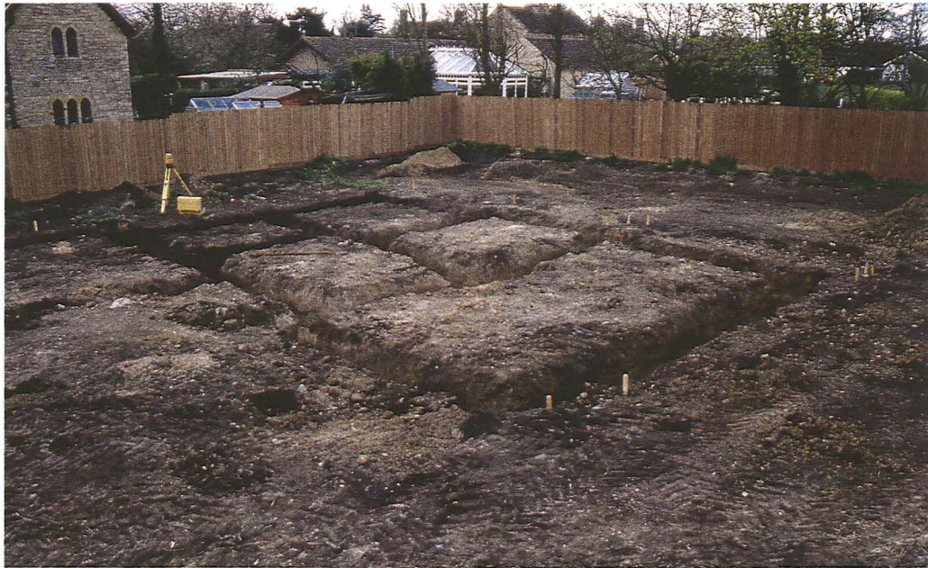
Plate 1 General view of excavated foundation trenches for Plot 1
