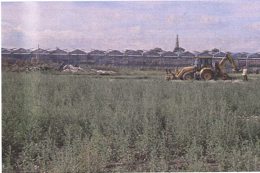
Plate 1 General view of site, looking south
