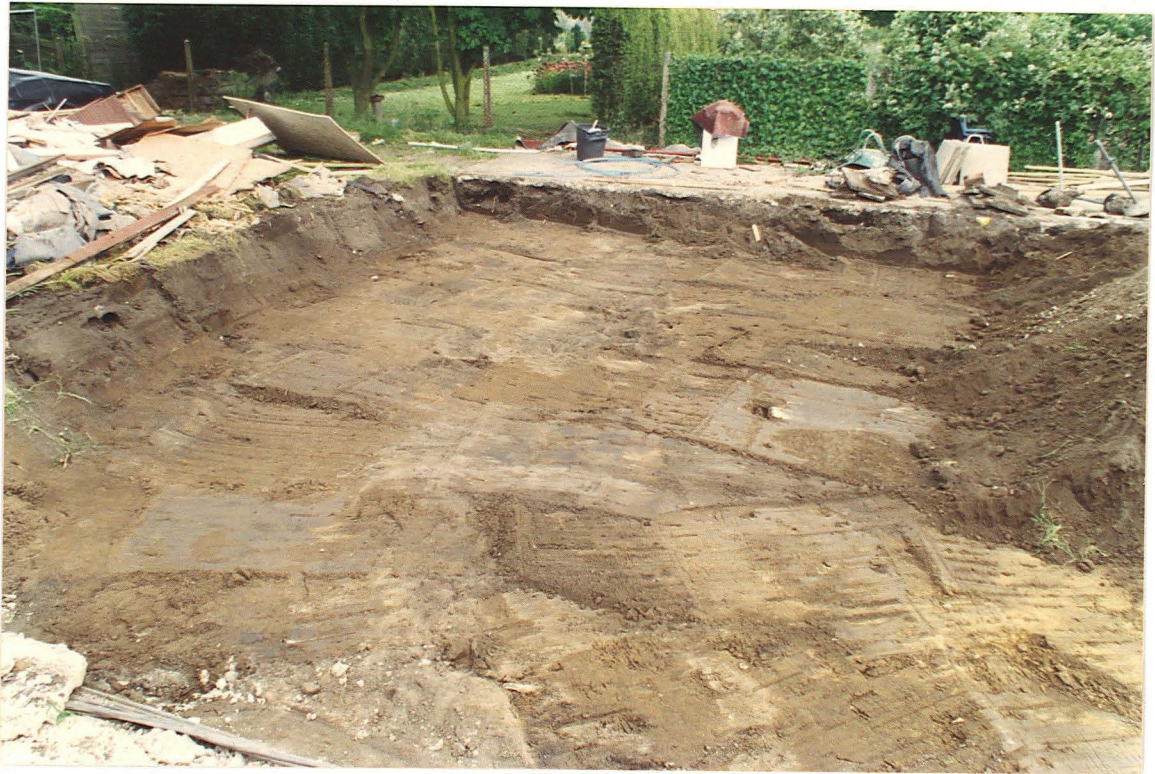
Pl. 3 Topsoil stripping in progress at west end of area.
