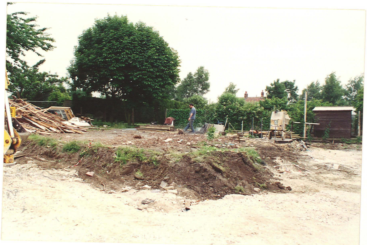
PI. 2 Proposed car park showing area after removal of temporary building and prior to reduction in height. Note foreground where ground has already been reduced to required level and stoned.
