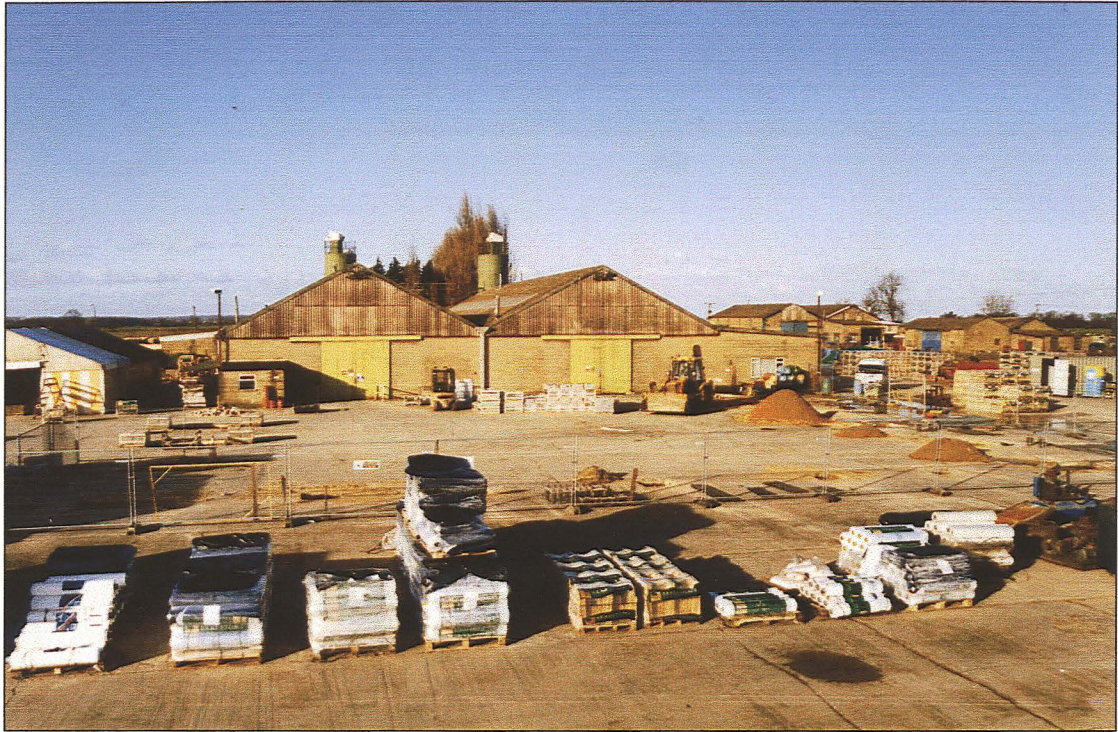
Plate 1 Site location showing excavated pits
