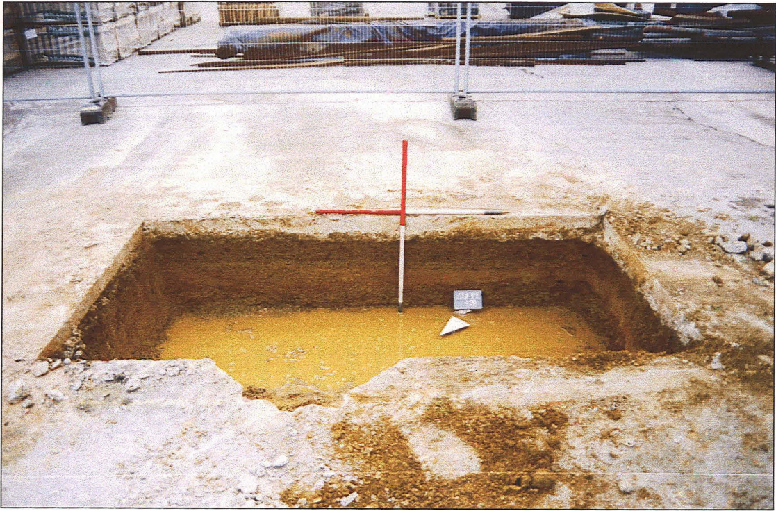
Plate 3 Foundation pit 5 showing layering of natural deposits below the concrete platform
