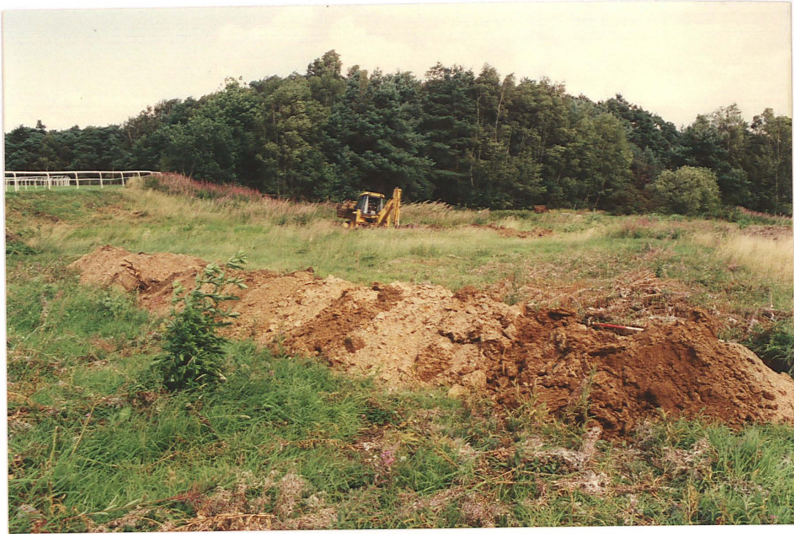
PI. 5 Location of Trenches 2 and 3. Looking north east.
