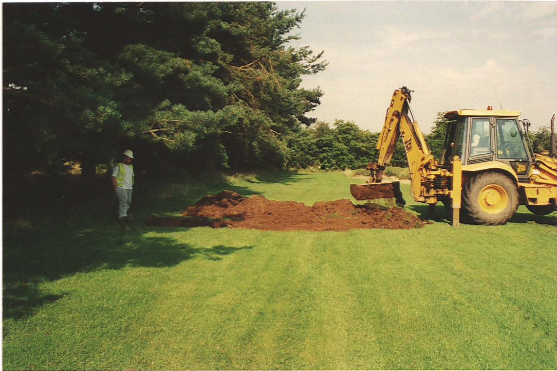
PI. 1 Archaeological monitoring of topsoil stripping.
