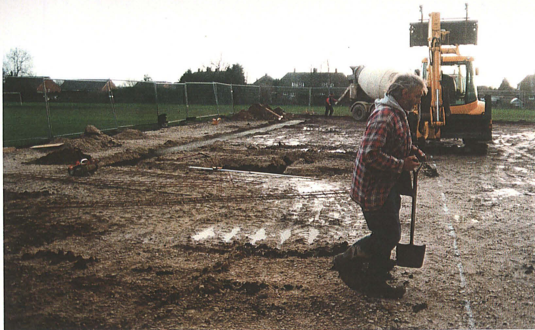
P1. General view of groundworks looking south
