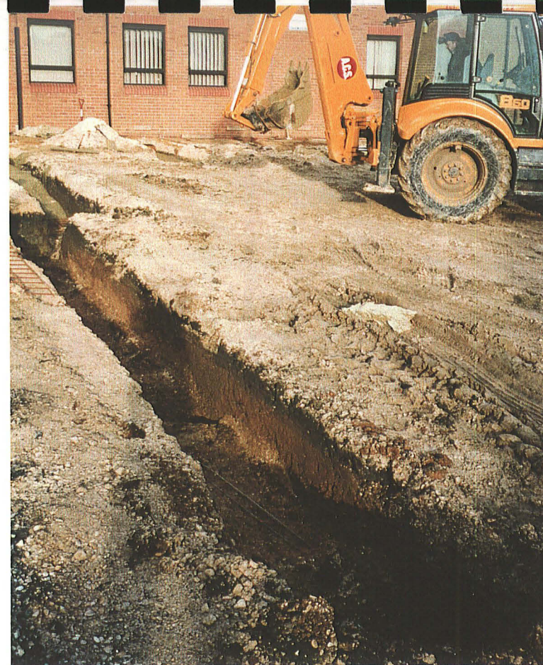
P2. Features 018, 010 and 011 in west footing, looking north-east
