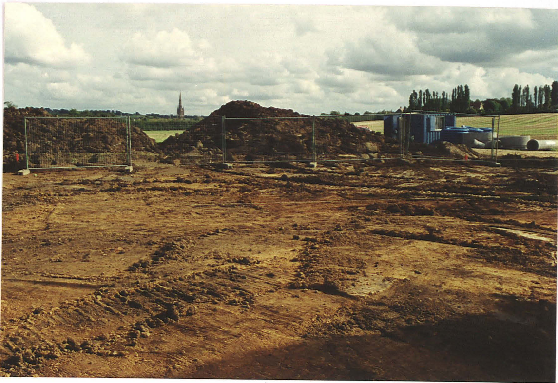
Pl. 1 Area topsoil stripped for the new pumping station (looking SE).
