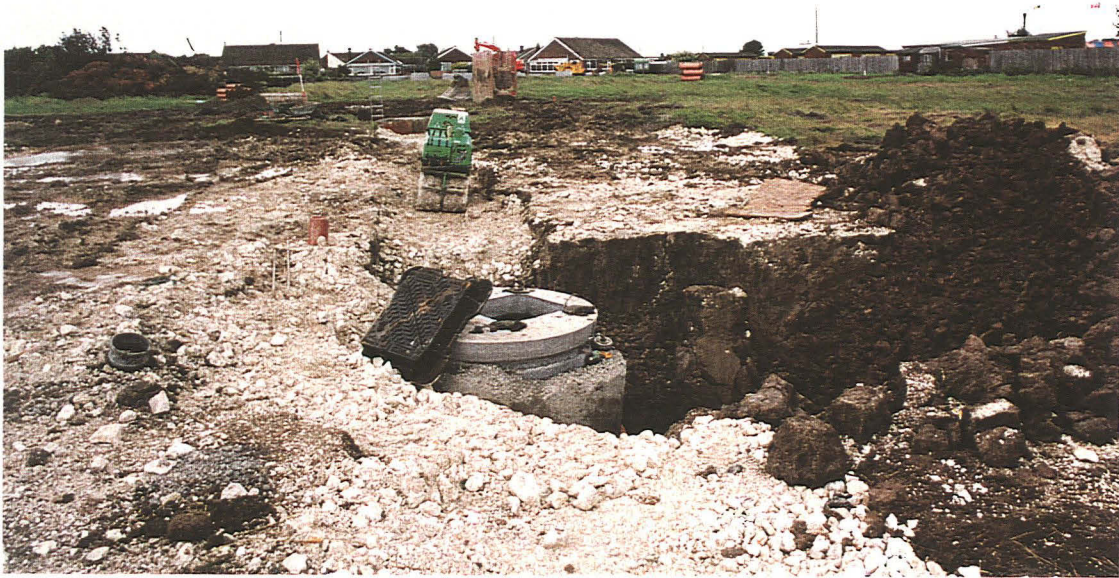
PL1: General shot of the site, looking north-north-west
