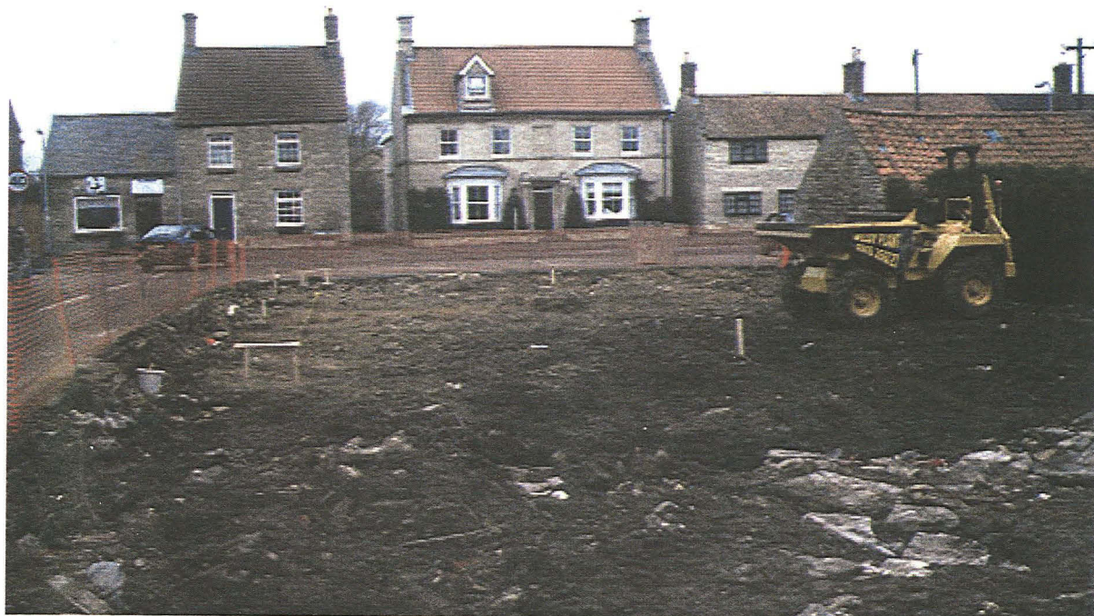
Plate 1 General view of site during excavation, looking west.
