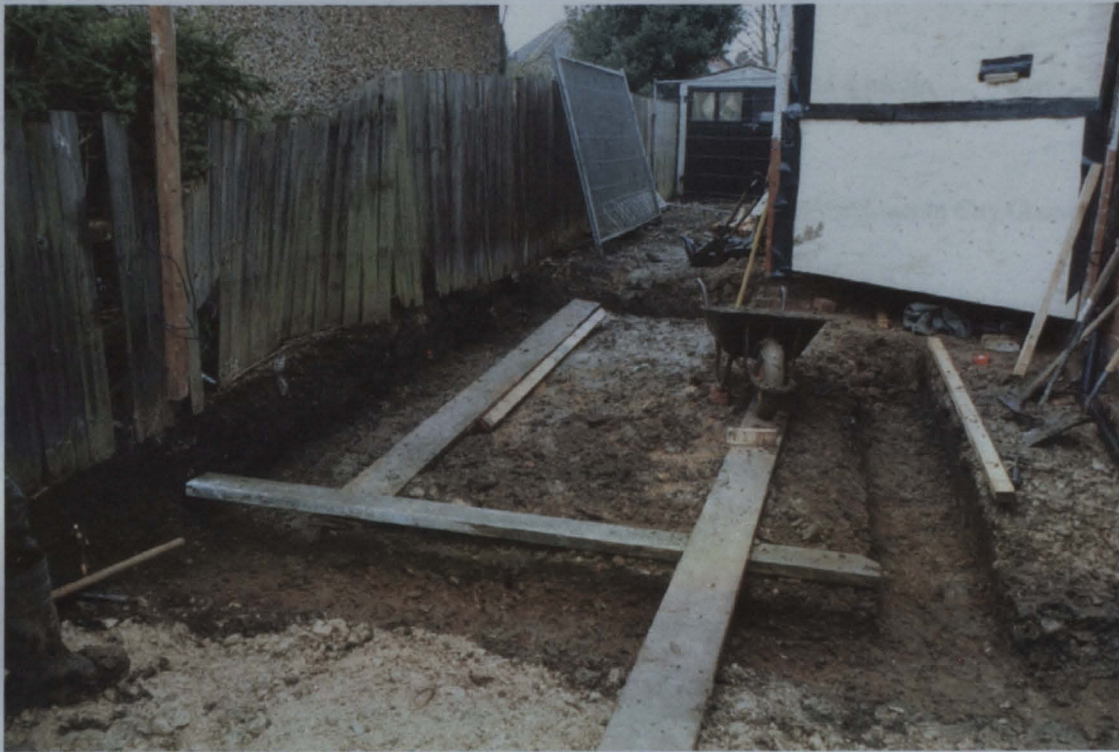
Plate 1: General view of foundation trench network - looking north
