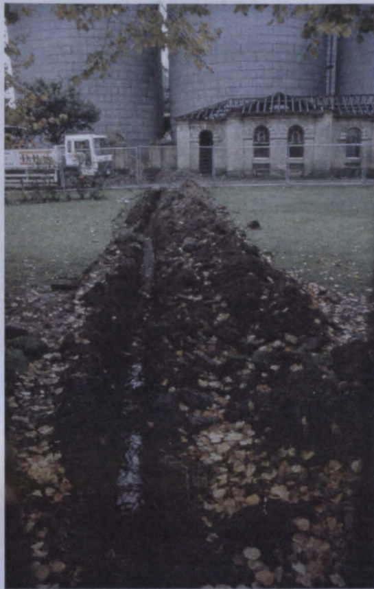
Plate 3 - View along the electricity cable trench, looking south
