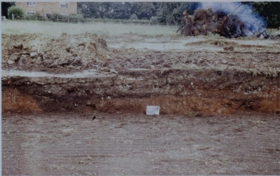
Plate 2 Section 1 in the terrace face, looking east.
