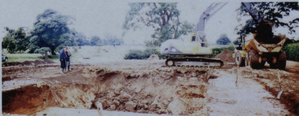
Plate 3 General view of the pool excavation in progress, looking west
