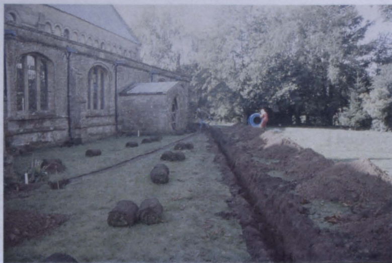
Plate 1 - View of the service trenches, looking southwest
