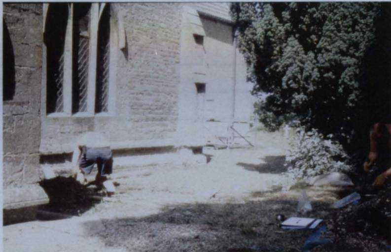
Plate 2 - General view of the southern drainage trench, looking northeast
