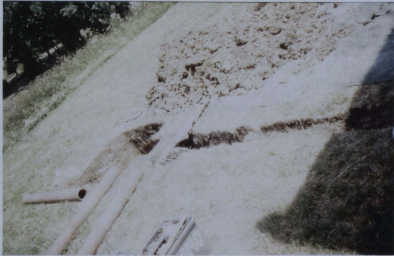
Plate 1 - General view of the northern drainage trench, looking northeast
