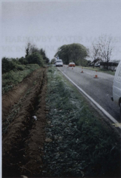
Plate 1 - The pipeline trench along Ermine Street, looking southwest
