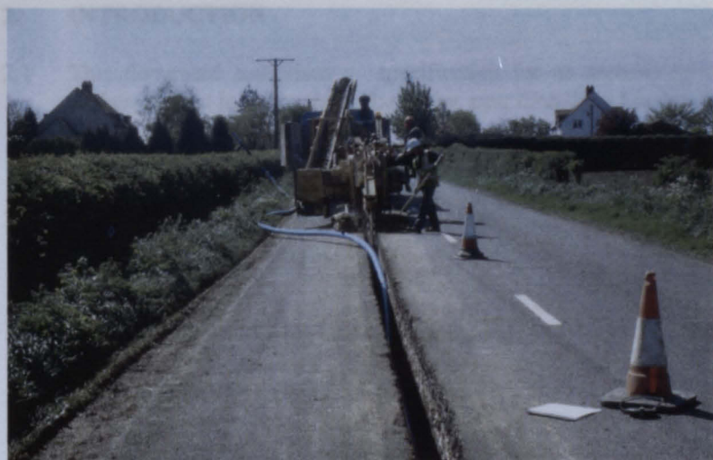
Plate 2 - The pipeline trench near Harrowby, looking west
