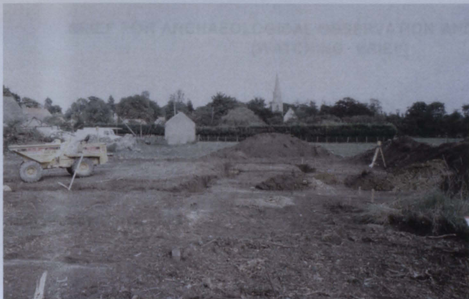
Plate 1 General view of the site looking east showing excavation of Plot 5.
