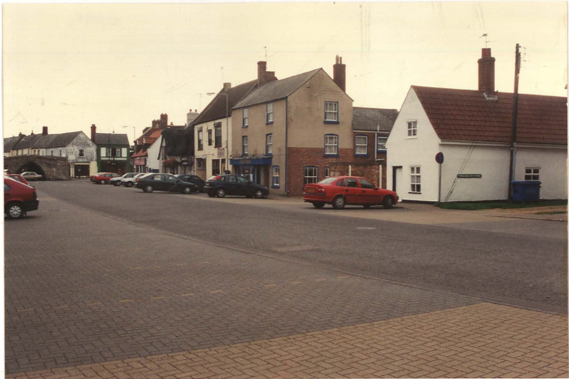
Pl. 1 North Street, Crowland, looking SE towards Trinity Bridge. Speechley's Yard is right foreground, with the blue shopfront of Frydays, 10 North Street, in front of the application site.
