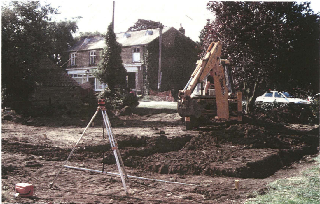
Plate 1 General view of site during groundworks, looking south
