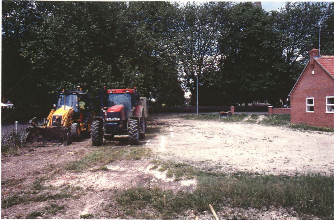
Plate 1 General view of site prior to groundworks
