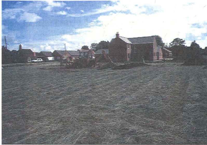
Plate 1 - General view of the development area, looking northeast
