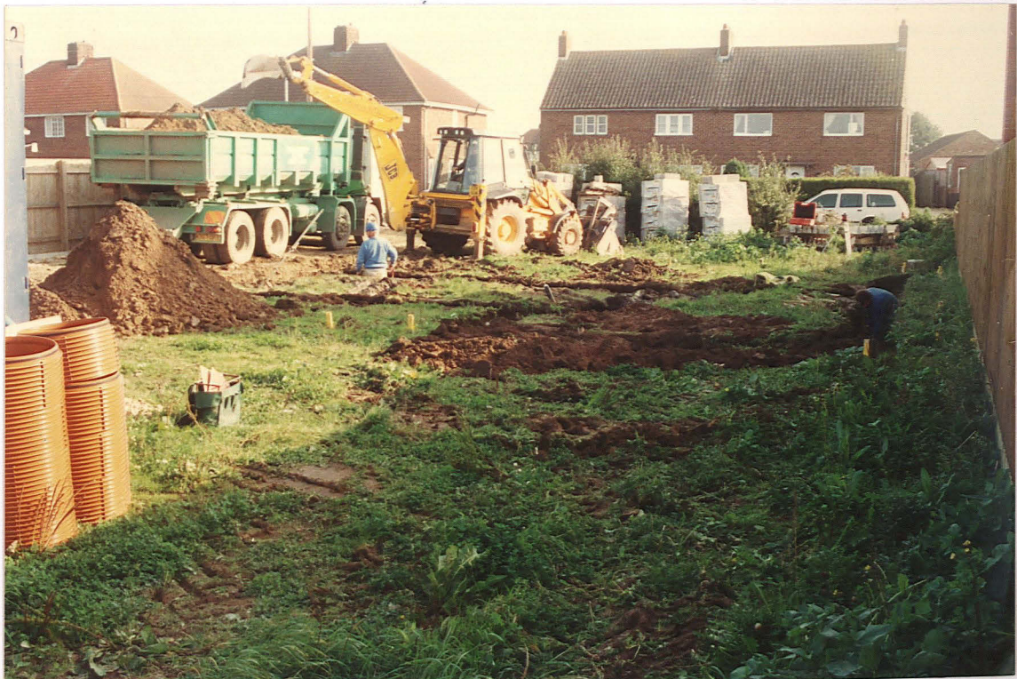
Pl. 2 Excavation of foundation trenches for Plot 5 (looking east to Drury Lane)
